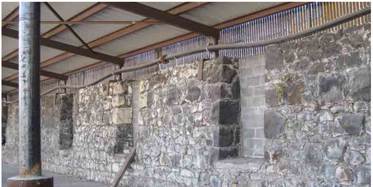
Woolen Mill basalt stone foundation walls
