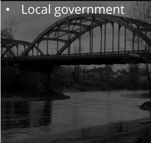
Image of Clackamas Bridge. Source: creative commons
