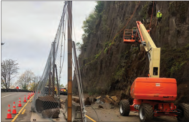
An example of rock scaling work to reduce the risk of rocks falling on a roadway.
