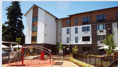
Terrace Glen Apartments in Tigard was funded by Metro’s Affordable Housing Bond.
