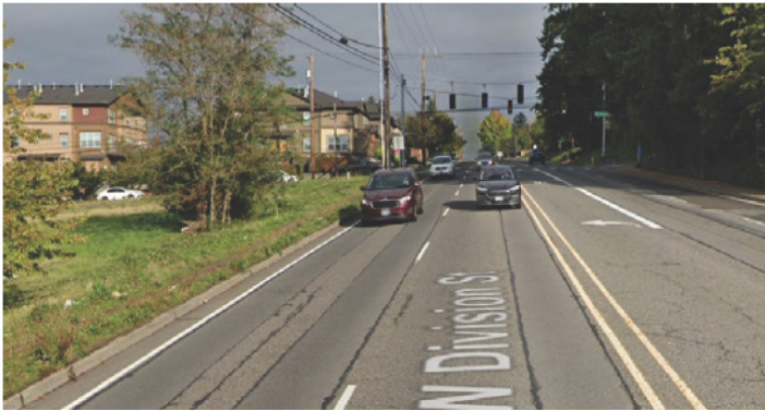
NW Division Street - north side sidewalk gap
