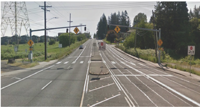
NW Division Street & Gresham-Fairview Trail Crossing
