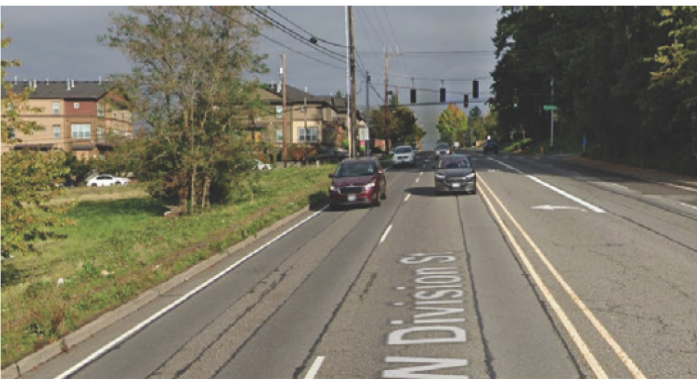
NW Division Street - north side sidewalk gap
