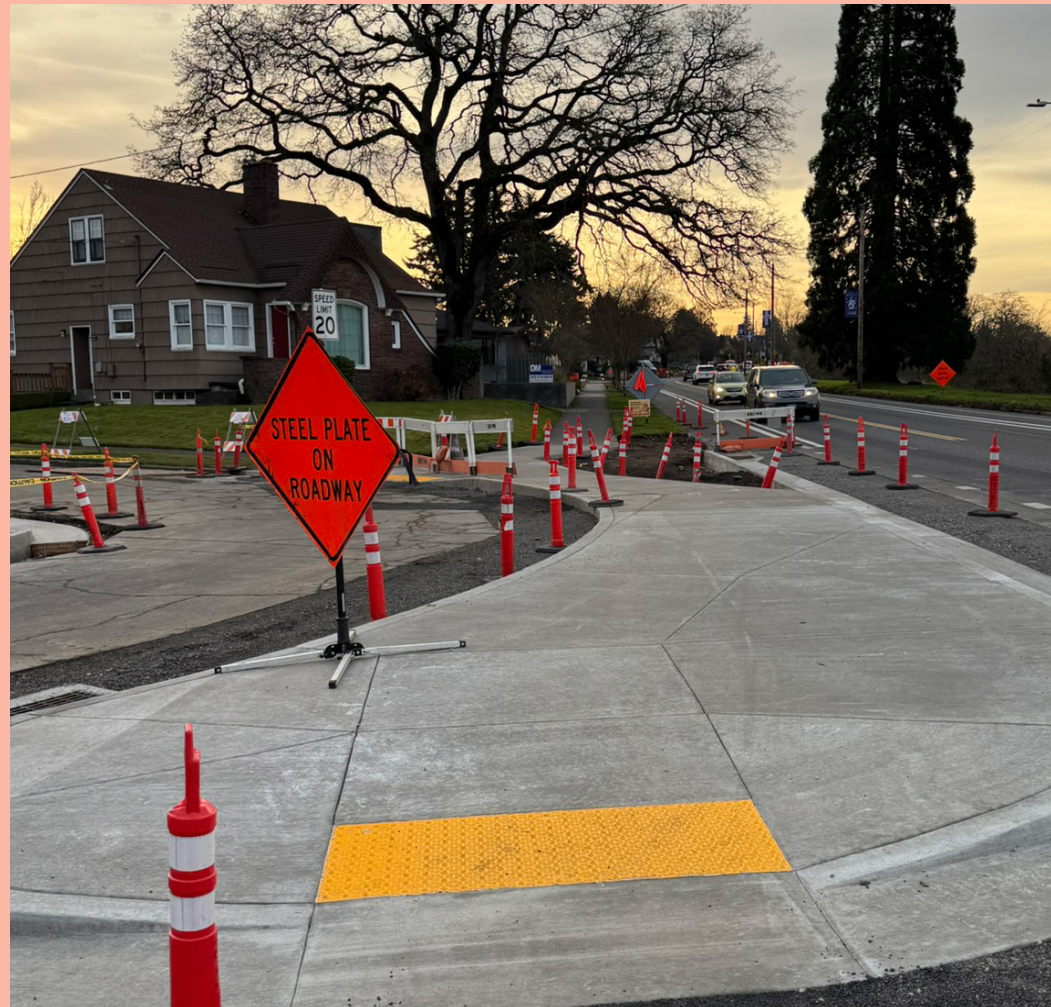
The 2027-30 MTIP includes number of project investments to build new compliant curb ramps to meet the Americans with Disabilities Act requirements.
