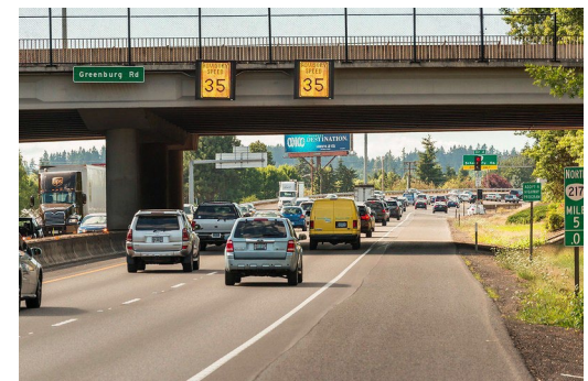
Example of variable speed signs on OR 217
