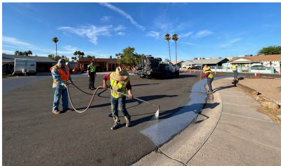
Figure 23. City of Phoenix crews applying a reflective coating to a street as part of the Cool Pavement Program.
