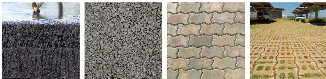
Figure 21. Examples of porous asphalt (left), pervious concrete (middle left), interlocking pavers (middle right), and P-ACBs (right).
