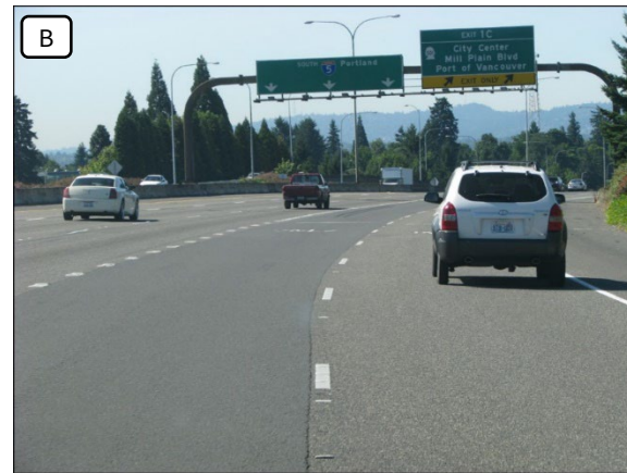
Southbound I-5 at Mill Plain Boulevard off-ramp auxiliary lane
